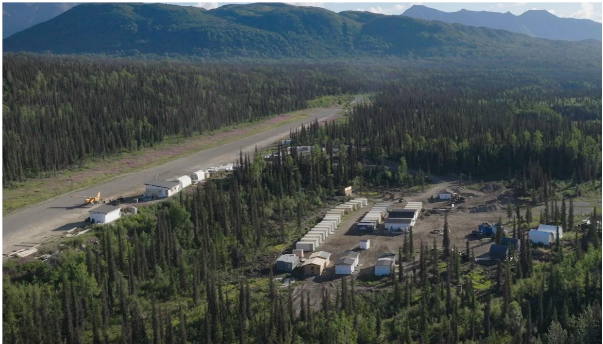
Figure 4-3: Aerial view looking north of the Whiskey Bravo airstrip and the Estelle 80-person winterized camp and facilities
