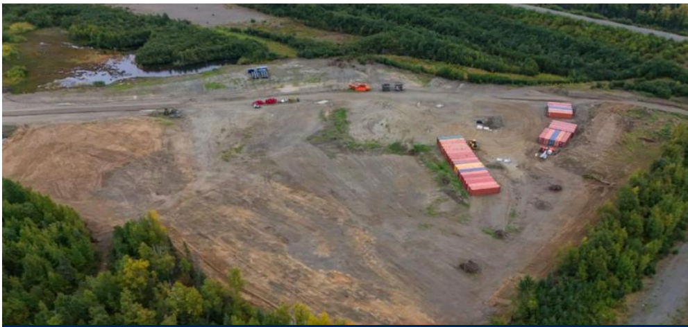
Antimony processing plant site which has been prepared ready for construction
