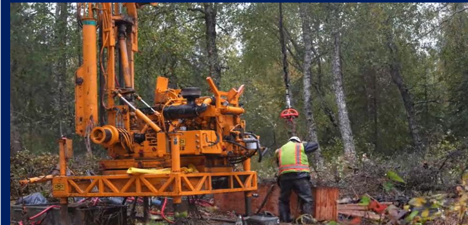
Geotechnical drilling on the West Susitna Access Road route
